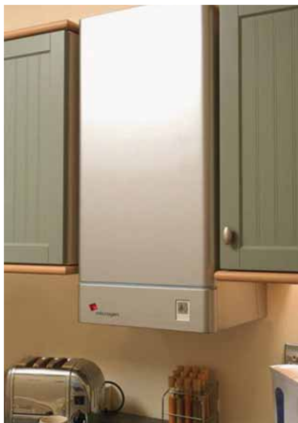
Wall-mounted Microgen Appliance installed in kitchen
