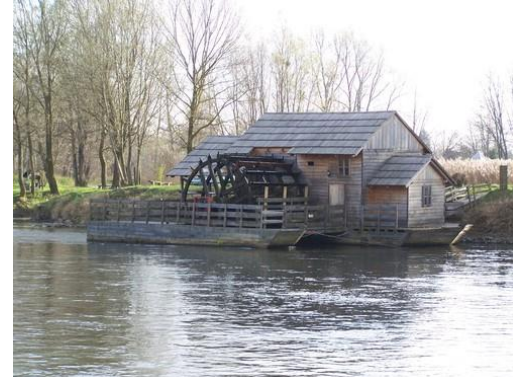
(c) Replica floating mill in still in operation on the Mura river in Croatia
