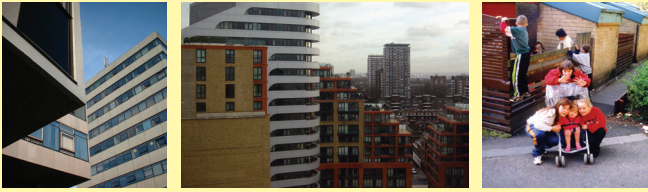
Fig.1 to Fig.3 A significant fraction of the UK building stock will require refurbishment within the next few years in order to meet peoples' demands for a good quality of life.
