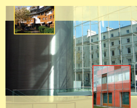
Fig.9 Examples of the three identified building envelope types: Single skin envelope, double skin envelope and climatic envelope
