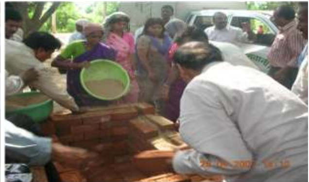
CAVITY FILLED WITH SAND
