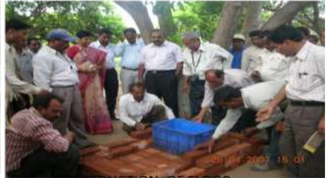
CONSTRUCTION OF FLOOR
