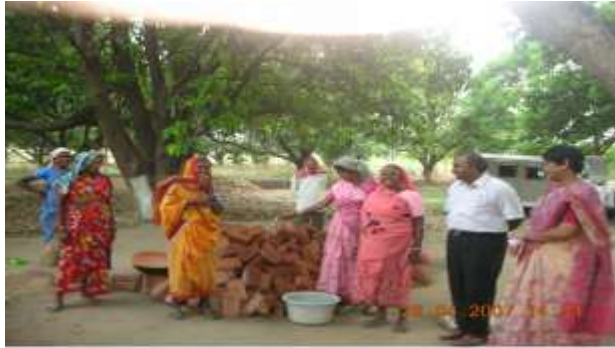
WATERING OF BRICKS
