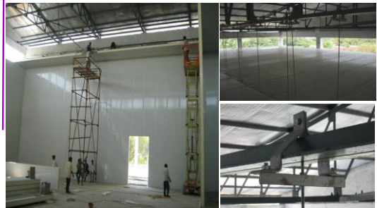
FIXING OF CEILING PANELS
