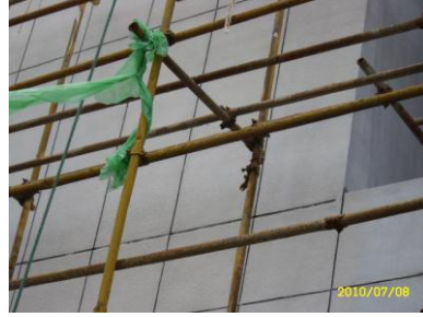
WALL INSULATION WITH PUF/PIR (EXTERNAL) FINAL FINISH
