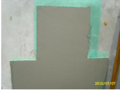
WALL INSULATION WITH PUF / PIR SLABS APPLICATION OF TOP COAT
