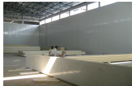
WALL PANELS ERECTED
