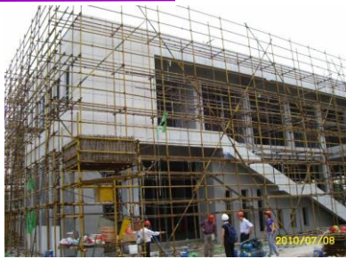
WALL INSULATION WITH PUF/PIR (EXTERNAL) FINAL FINISH
