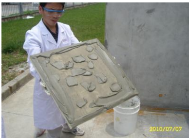
WALL INSULATION WITH PUF / PIR SLABS APPLICATION OF ADHESIVE
