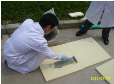
WALL INSULATION WITH PUF / PIR SLABS APPLICATION OF PRIMER COAT
