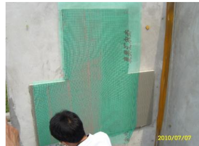
WALL INSULATION WITH PUF / PIR SLABS FIXING OF REINFORCEMENT MESH
