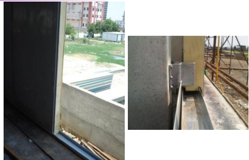
PANEL FIXING ON FLOOR WITH CHANNEL
