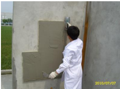
WALL INSULATION WITH PUF / PIR SLABS APPLICATION OF BASE COAT
