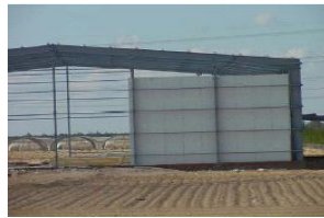
FIXING OF HORIZONTAL PANEL FROM INSIDE CA STORAGE
