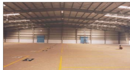
LARGE CLEAR SPAN
