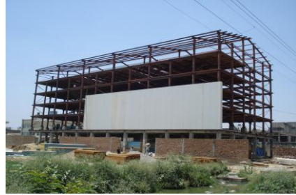
VERTICAL FIXING OF PANELS
