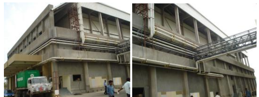
COLD STORE OVER EXISTING RCC BUILDING COLD STORES
