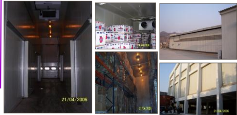
PEB & PANELS, RCC COLUMNS
