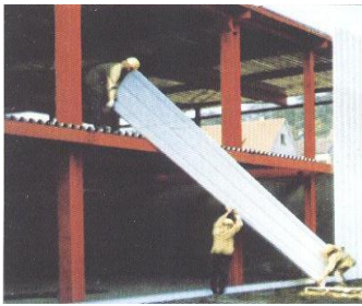
Lifting of panels for Wall
