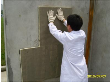
WALL INSULATION WITH PUF / PIR SLABS FIXING OF SLAB ON TO THE WALL
