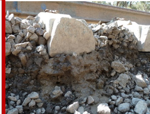
BALLAST DEGRADATION
