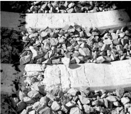
CRACKED SLEEPERS
