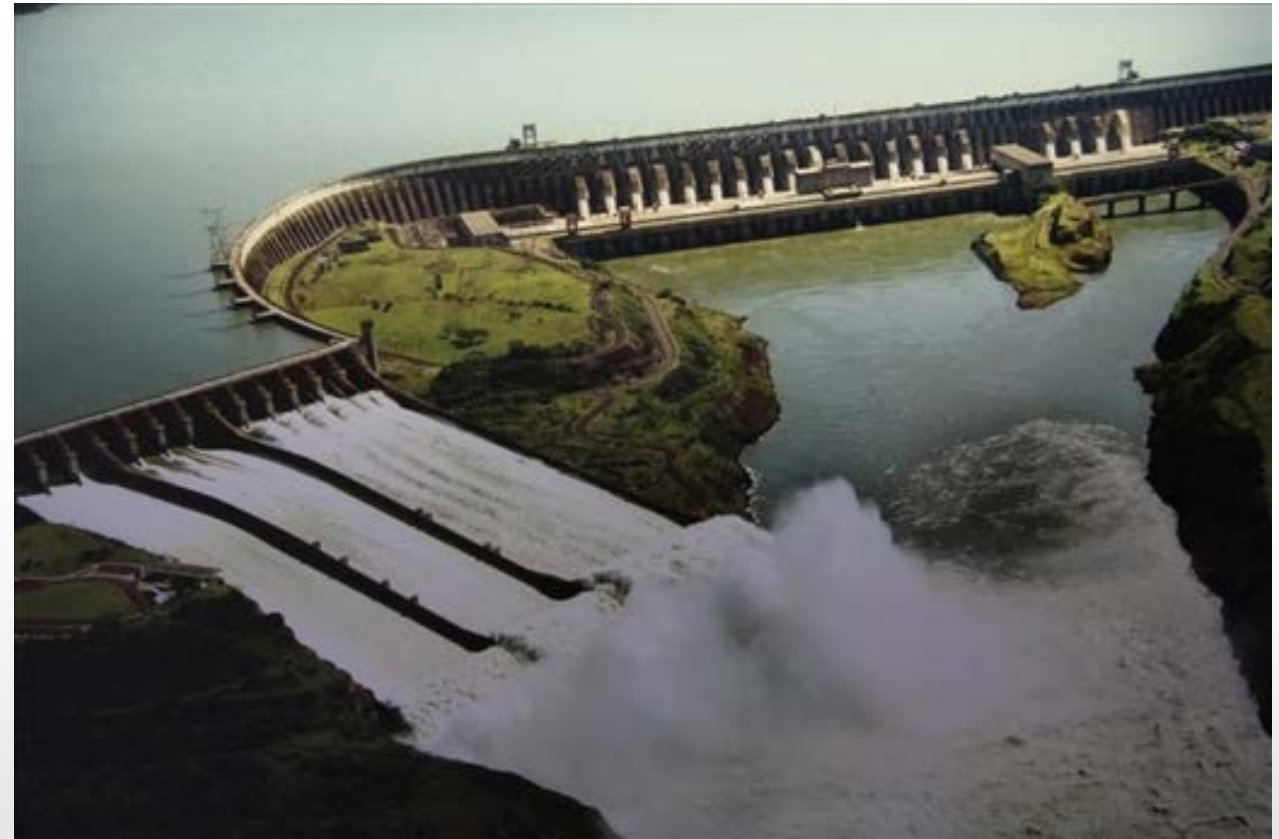
Figure 1: Itaipu Hydropower Dam, Brazil. Source: https://journals.worldnomads.com/
